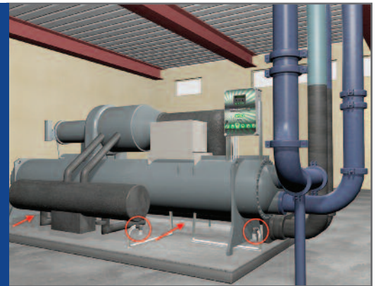
Typical installation. Multiple sampling points surround the chiller for maximum protection.
